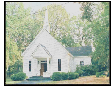
Pictured is the Andersonville Baptist Church building after exterior repairs and painting.
